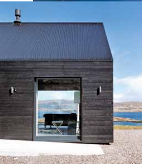
above HardiePlank exterior cladding covers the entire property; it's an Australian system (concrete composite siding) that is durable and will never need painting
